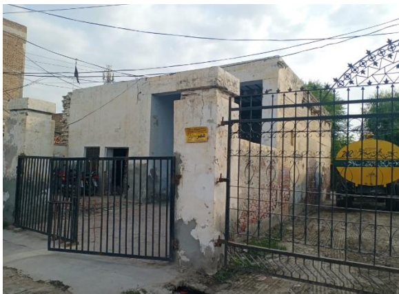
Figure 24: Front view of Fire Brigade
