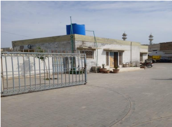
Figure 32: Front View of Audit Branch & Work Shop
