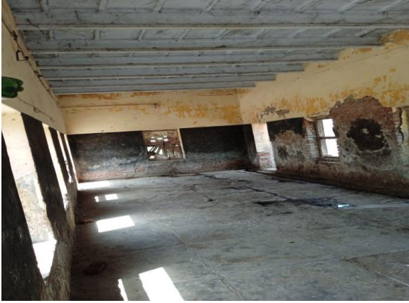
Figure 28: Front View of the Slaughterhouse
